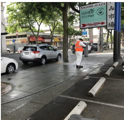
Crews pressure washed
